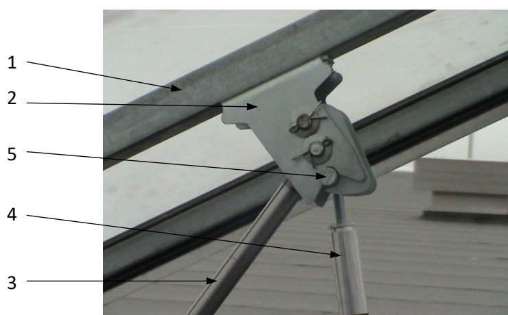
Fig. 21 Mechanical hook lock
